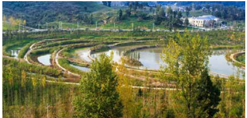
Terraced bio-swales on steep slope
