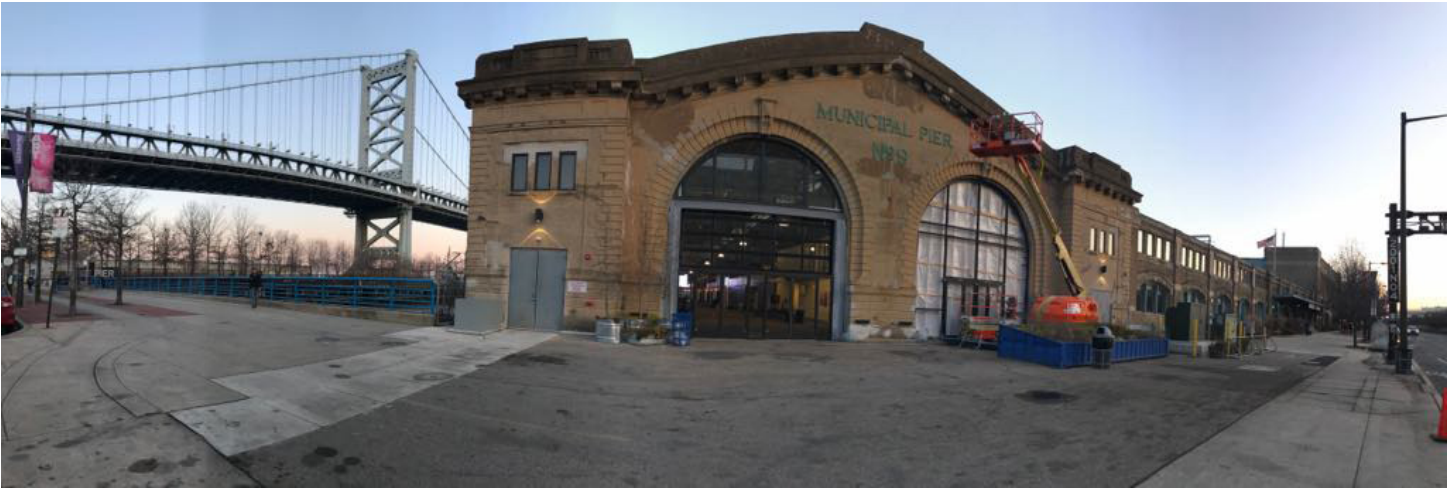
Front entrance view of Municipal Pier No. 9
