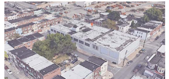
Existing Conditions: View From The South West
