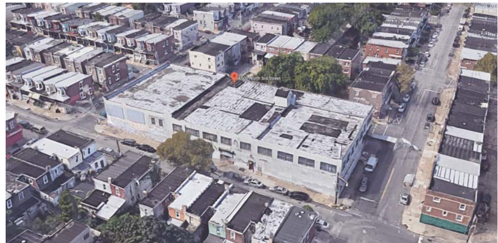
View of North East Corner
