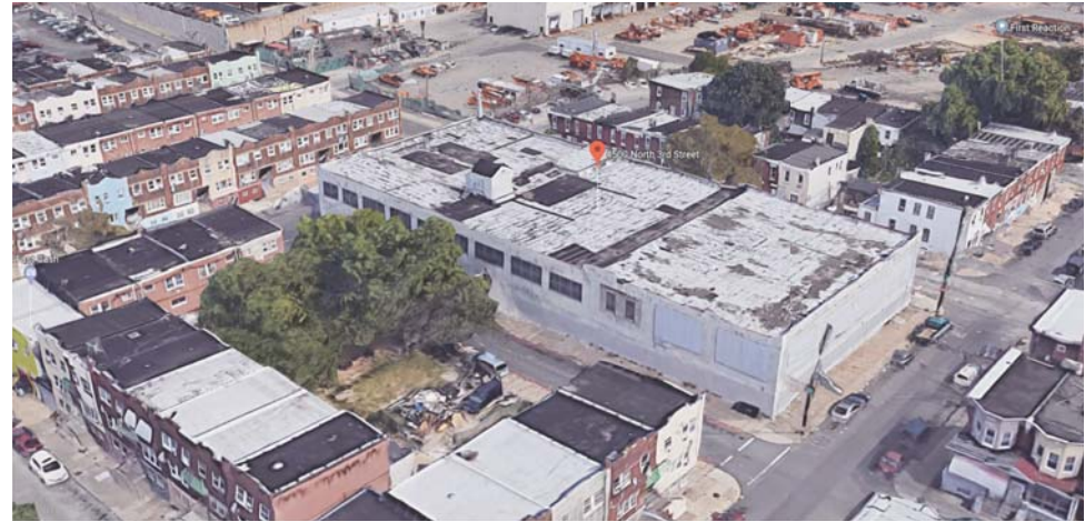
View of South West Corner
