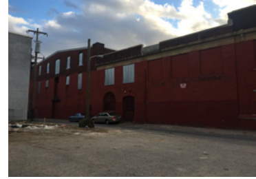
Outdoor Site West View
