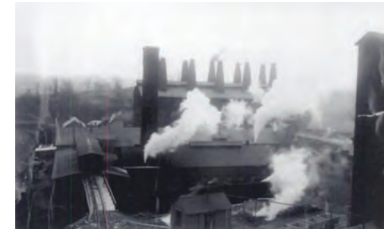
COPLAY CEMENT MILL B
