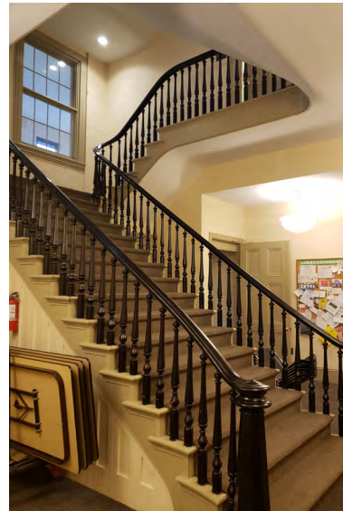
EXISTING CENTRAL STAIRCASE
