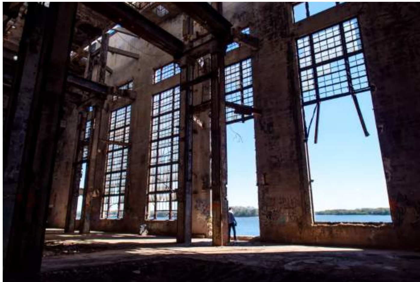
INTERIOR CONDITIONS - Abandoned
