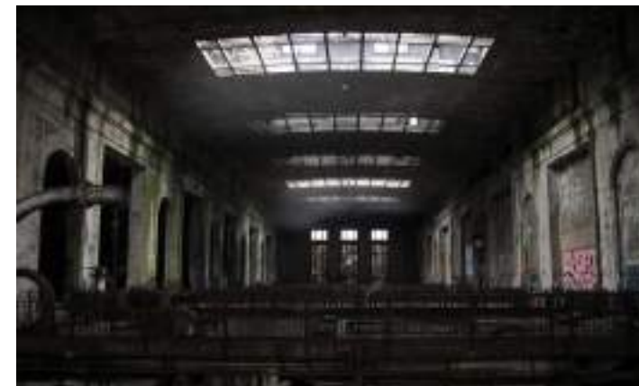
INTERIOR CONDITIONS - Abandoned
