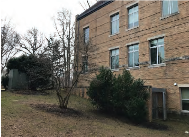
East Facade - to understand slope
