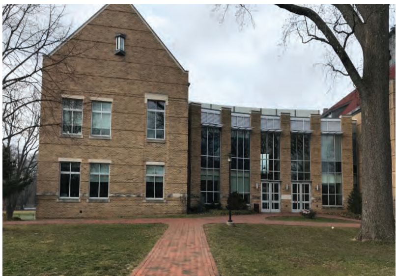
South Facade - existing 2nd floor entrance
