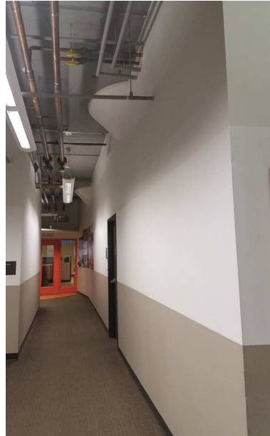
Inset Concrete Mushroom Columns in 1920 Wing
