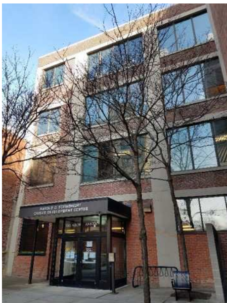
Building Courtyard Steinbright Career Center Entrance Looking Northwest
