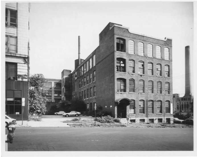
3201 Arch Street Circa 1975 Northeast view
