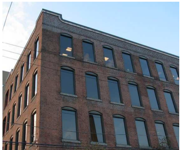
Building Window and Facade Detail, Southeast Corner Looking Northwest
