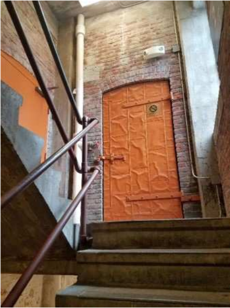
Original Fire Stair Doors in 1920 Wing
