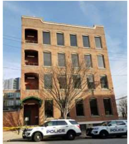
Building Entrance from Arch Street Looking North
