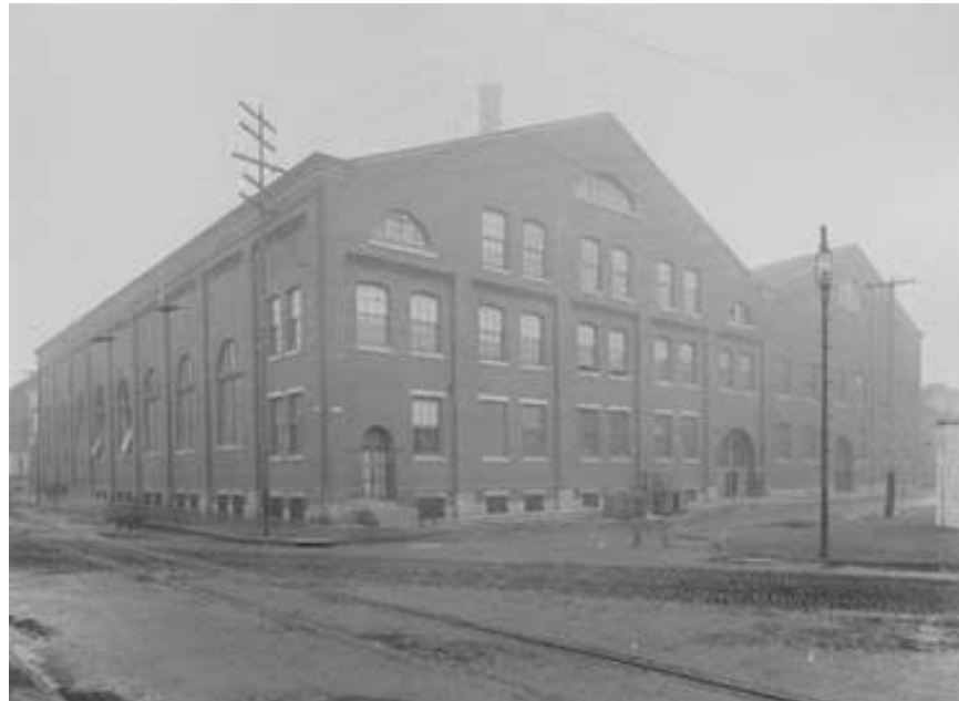
constructed in 1925 as a trolley repair warehouse
