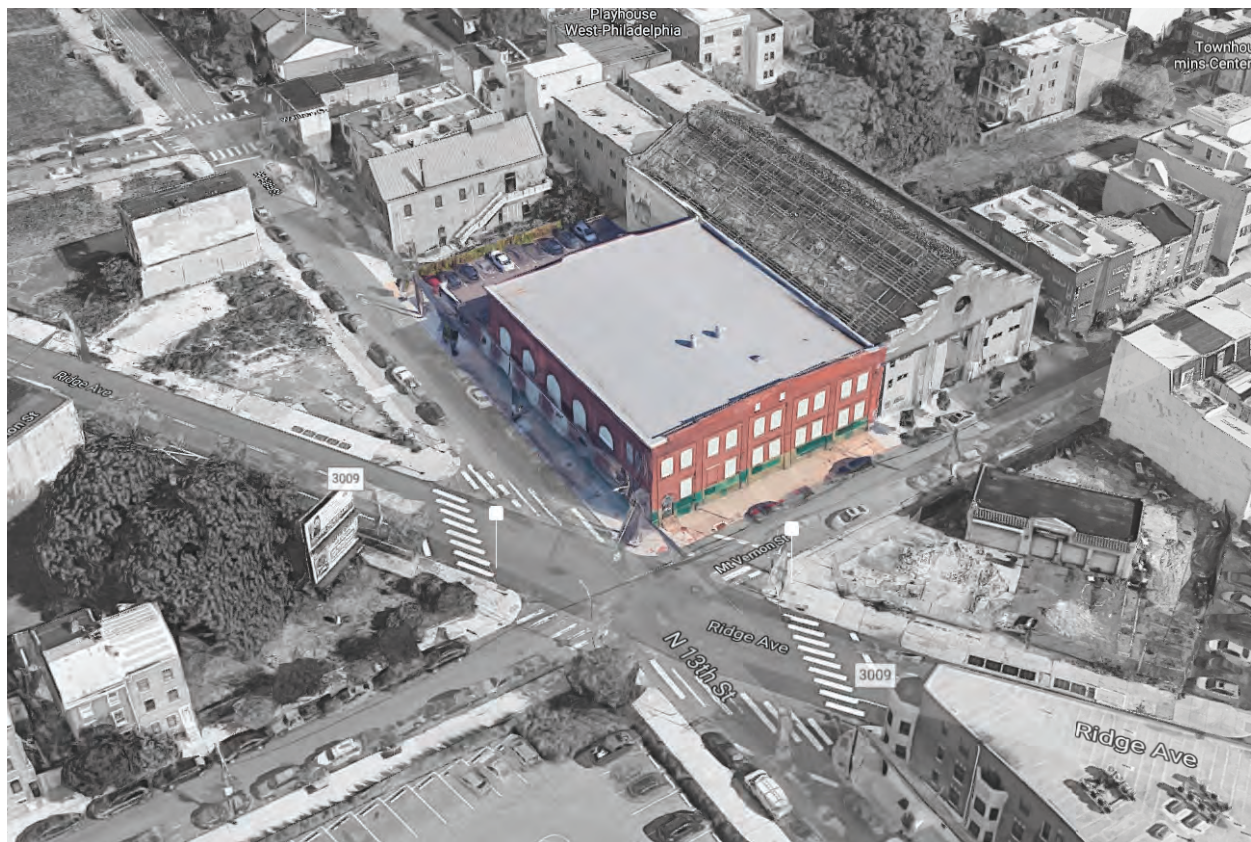
today the building is a SEPTA substation
