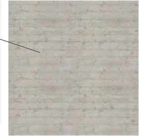
pale board-formed concrete infill
