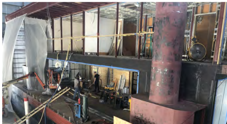
Construction of Deck
