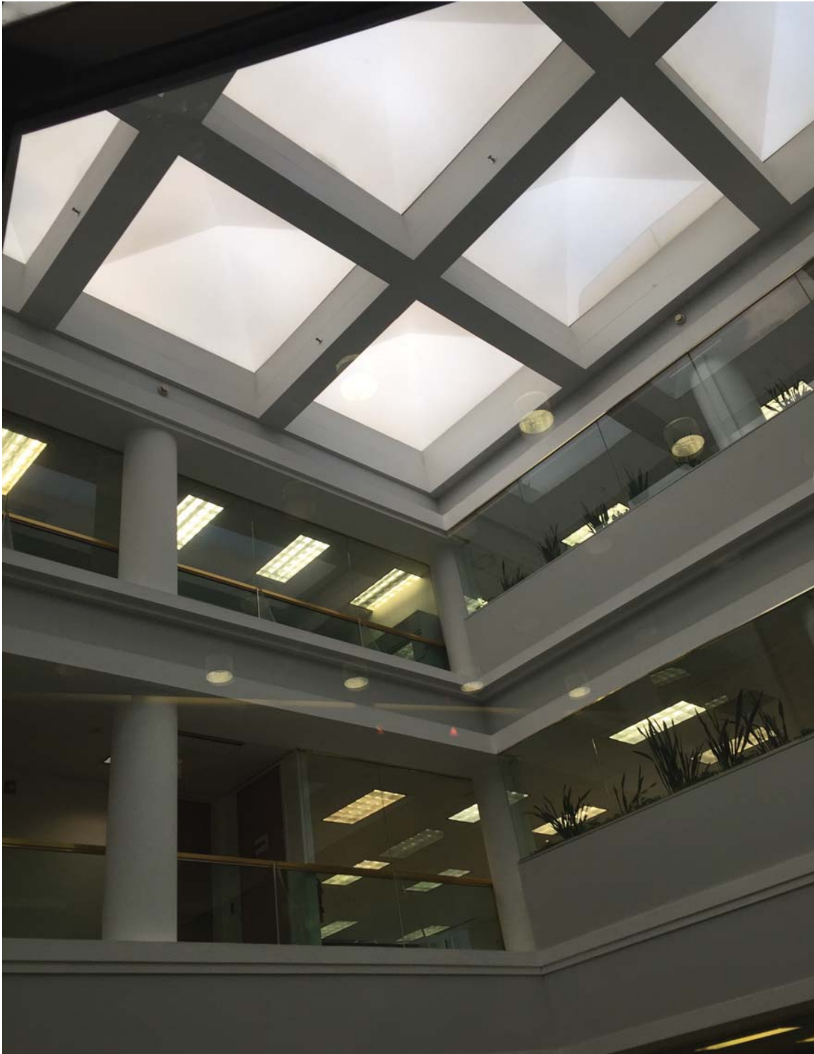
Image of the top of the atrium - from elevator.
