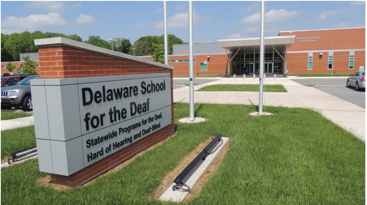
DSD EXTERIOR IMAGE
