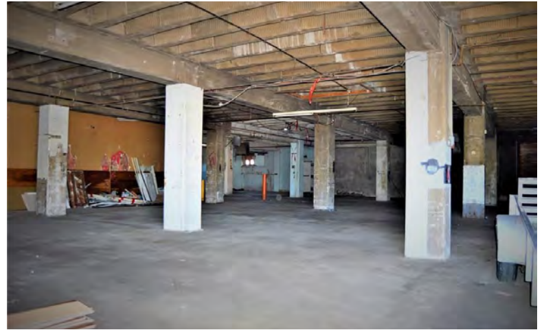
Interior view of the first floor and existing structure
