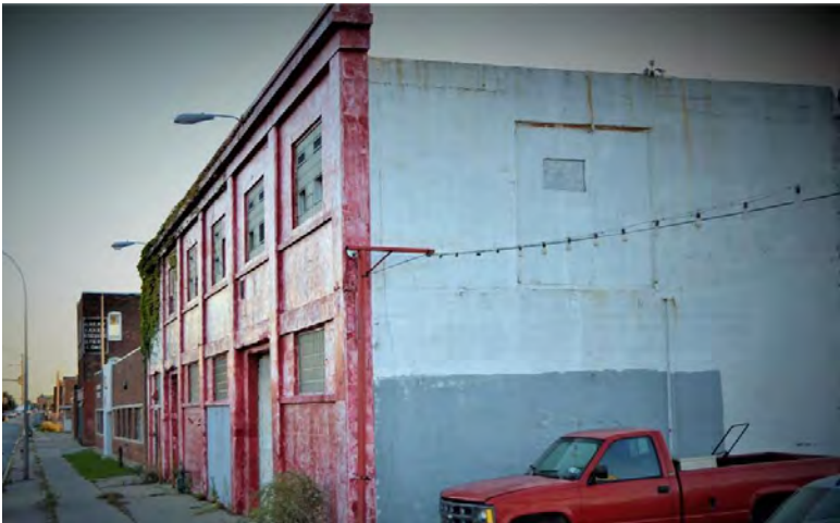
Exterior view of facade looking south down Niagara Street
