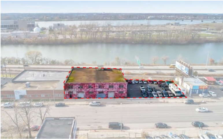
Bird's eye view of site looking west toward Canada
