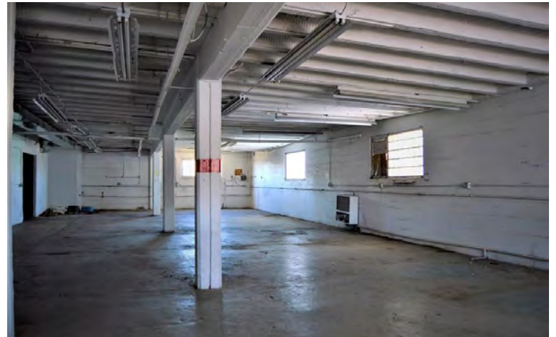
Interior view of second floor
