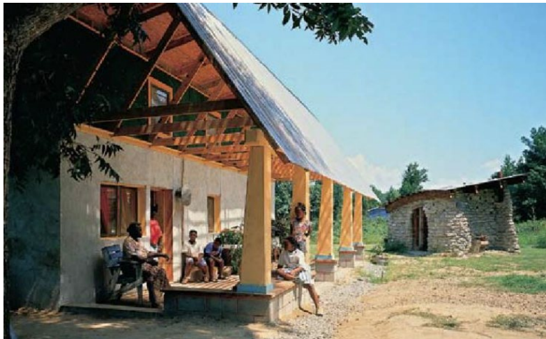
Figure 5: The rebuilt Bryant House, the first home completed by Rural Studio . Photograph by Andrea Oppenheimer Dean. Rural Studio: Samuel Mockbee and an Architecture of Decency. New York: Princeton Architectural Press.
