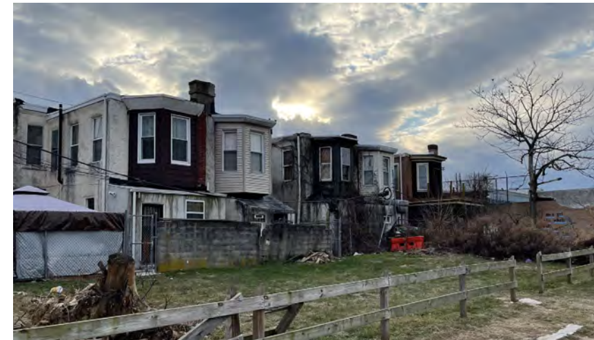
HARLAN STREET FACING SOUTH
