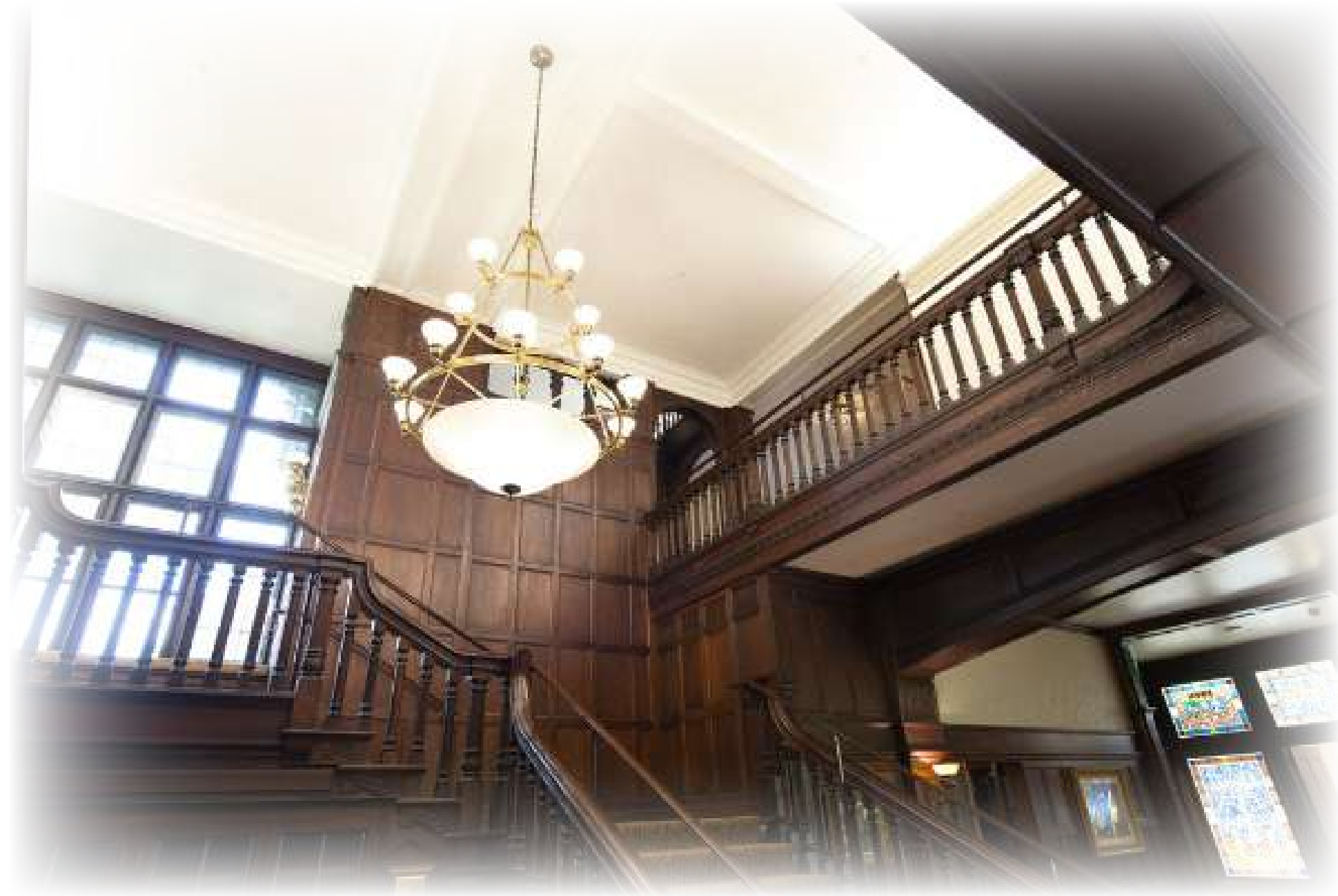
EXISTING MAIN STAIRWELL
