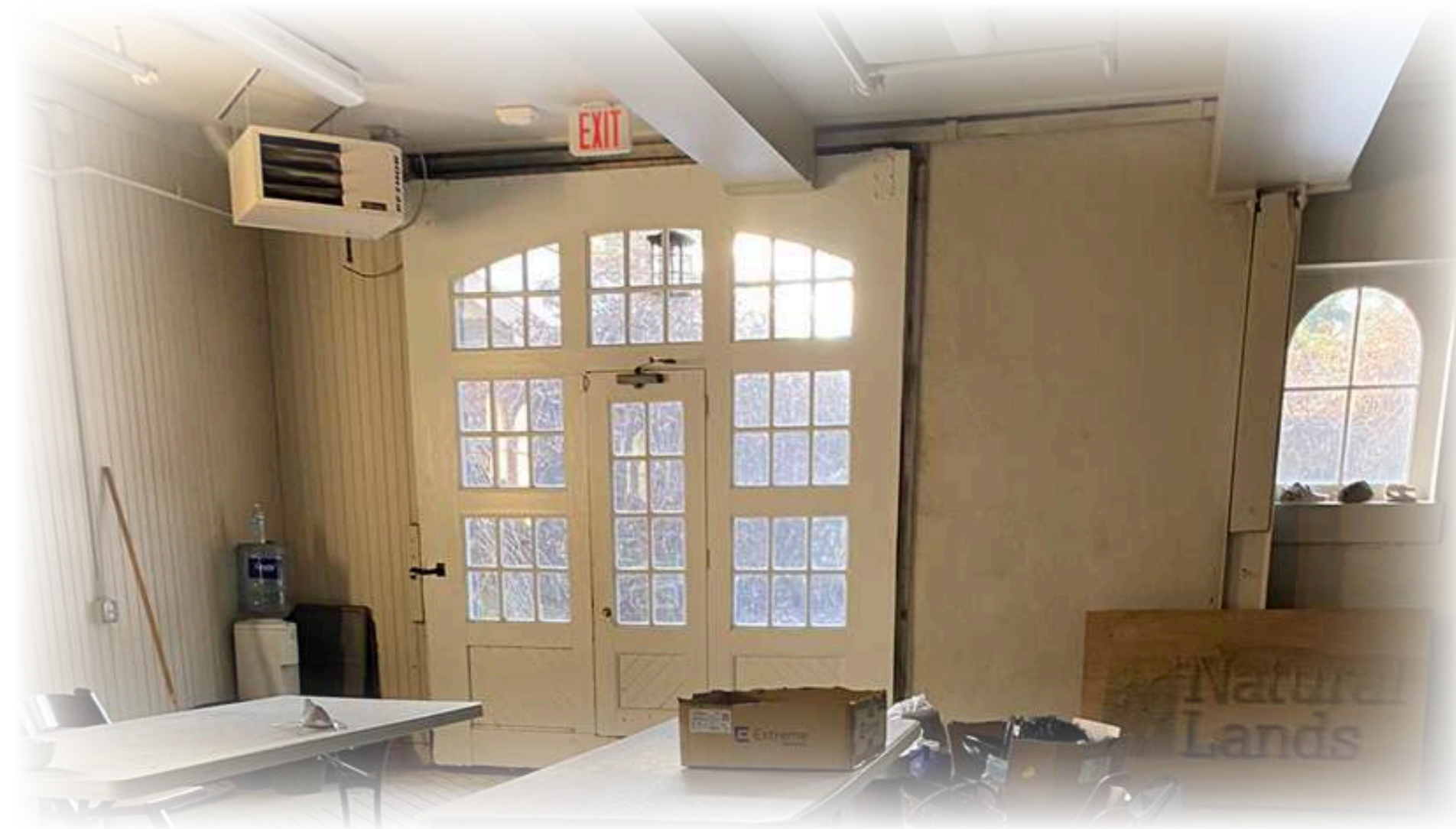
EXISTING WEST CARRIAGE BAY
