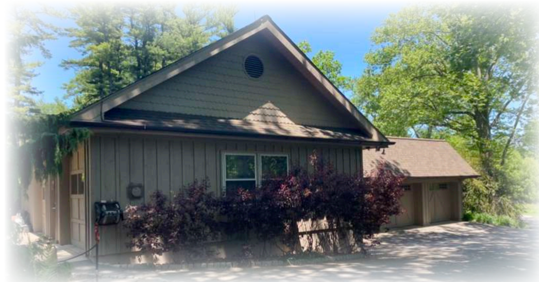
CARRIAGE HOUSE EXISTING GARAGE
